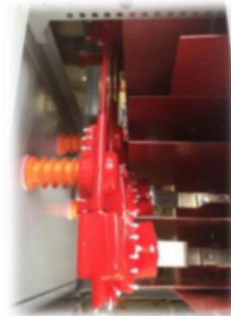
Figure 17: Optional Insulated Main Bus*
