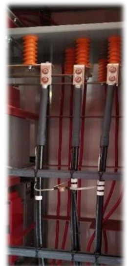
Figure 20: Load Take-Off Cable Connections*
