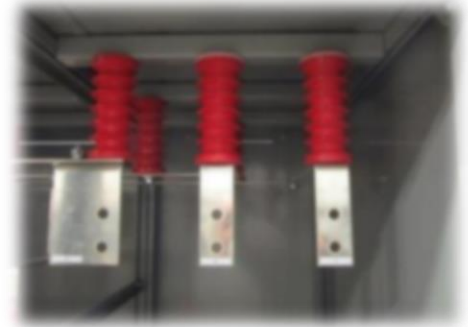
Figure 18: Load Take-Off Connection*
