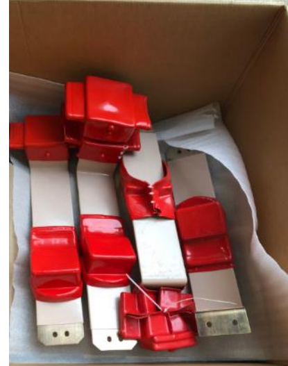
Figure 31: Ship Loose Switchgear Bus Splices for Contractor Installation During On-site Shipping Split Reassembly & Installation*
